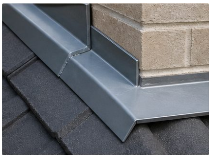
Main building roof assessment - Front roof elevation | Photo 1 Flashing detail - illustrative sample image; observations are supplied separately
